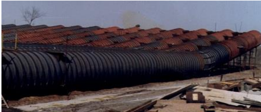
Cross drainage works carrying drainage over canal.
