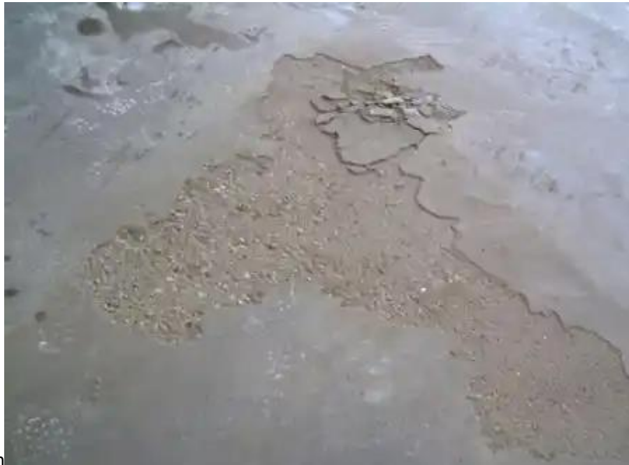
Fig 4: Delamination
