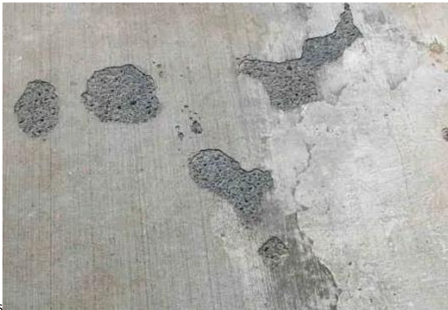
Fig 3: Concrete Blisters
