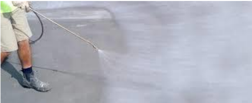
Fig.: Curing by the sprinkling of water
