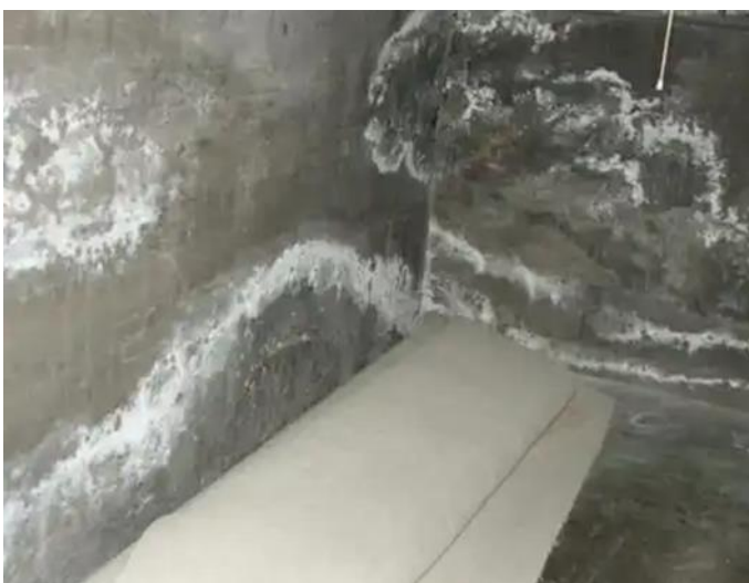
Fig 7: Efflorescence
