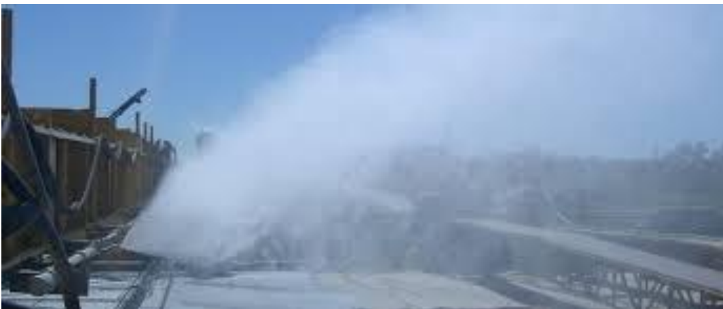
Fig.: Steam curing of concrete
