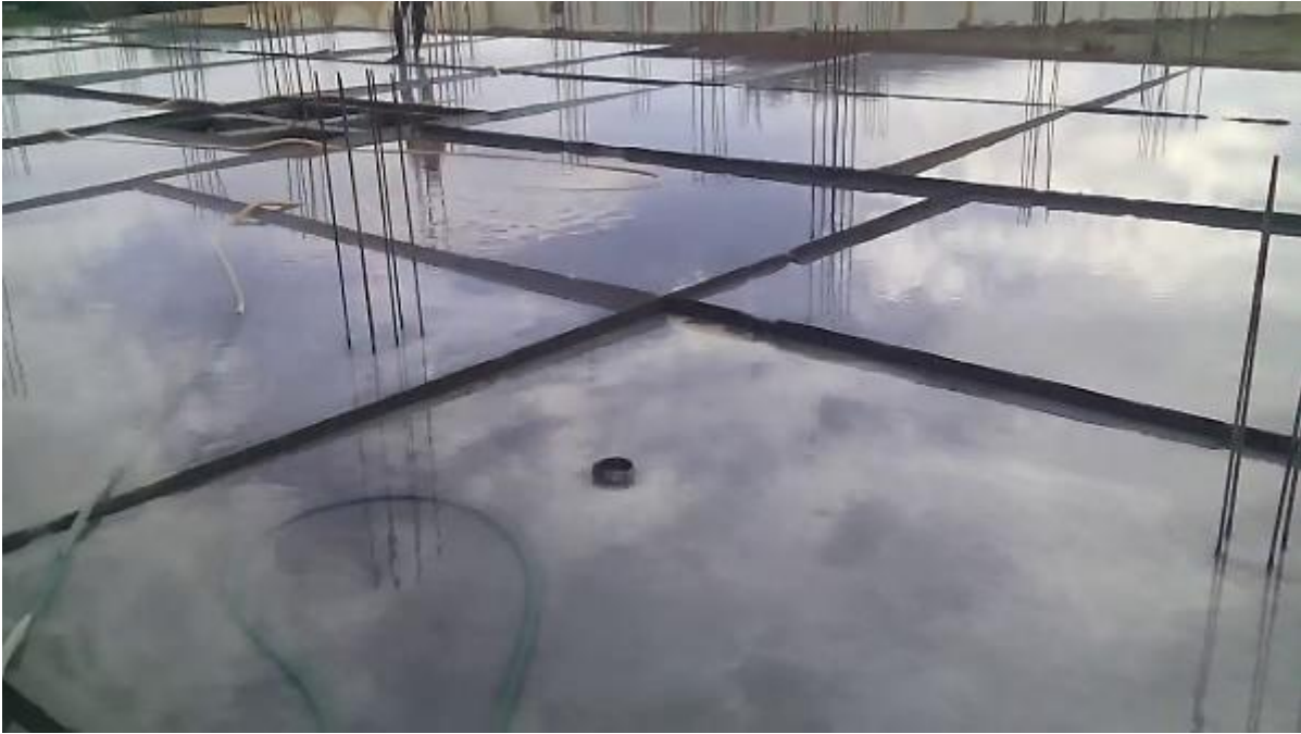
Fig.: Ponding of concrete
