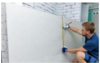
Plasterboard is a panel made of calcium sulphate dihydrate (gypsum) usually pressed between a facer and a backer. It is used to make interior walls and ceilings. This 'Drywall' construction became popular as a quicker alternative to traditional lath application.
